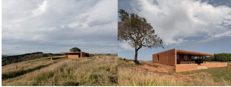
The decision to partially embed the architectural object —one meter into the ground— to shield it from cold winds also proved to be a smart solution for acquiring the key material for its construction: clay. This abundant local resource, renowned for its ceramic production quality, was essential for manufacturing modulated rammed earth panels directly onsite (Figure 8).
