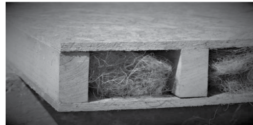
Fig. 3. Coconut fiber in wooden wall [14].
